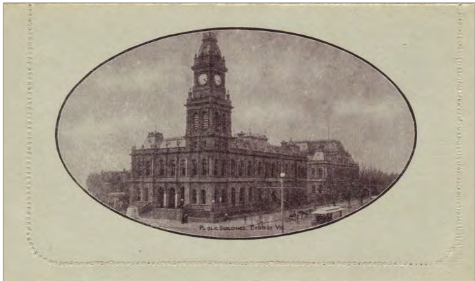
PUBLIC BUILDING BENDIGO VIC.
